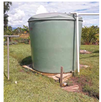
Replacement plastic water tanks are being installed to store rainwater for community use.
