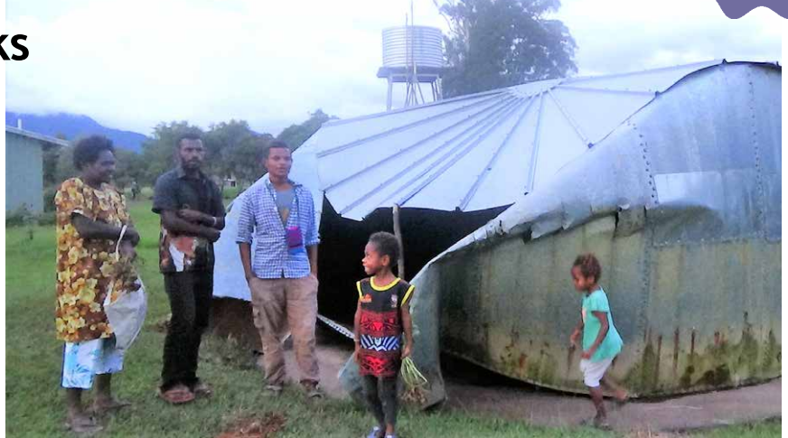
Collapsed water tank which served one of the student villages.
